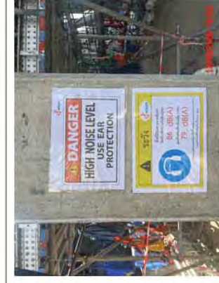
Picture 3 Warning sign installation around noise expose area
